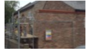
BRICKWORK TO EXTENSION
